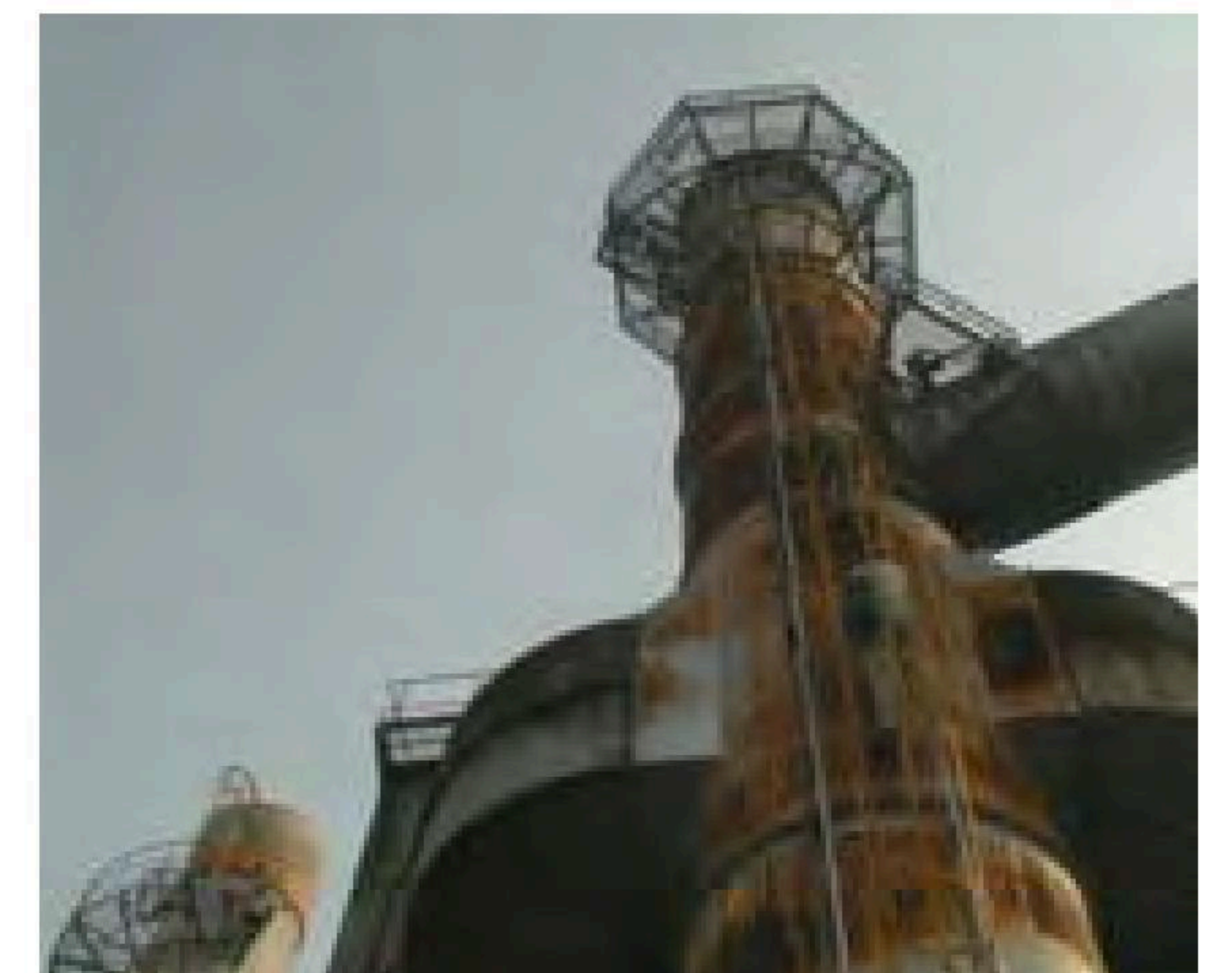
EP Exit Chimney
